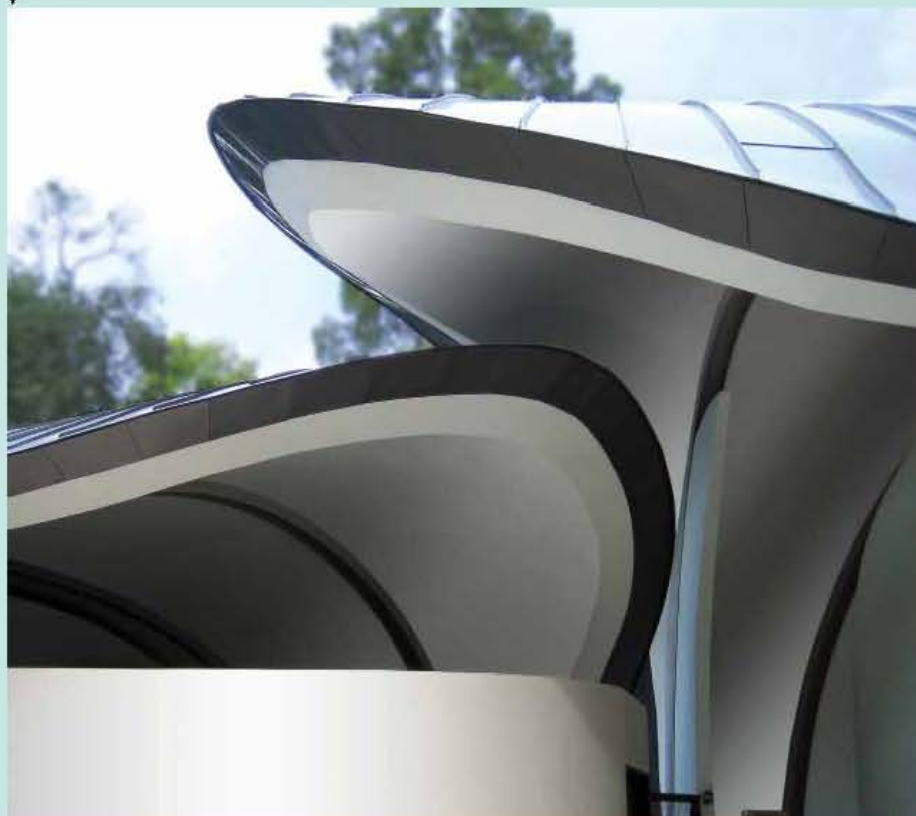
▲ The petal like form of the roof is constructed from free standing steel ribs that are expressed on the underside of the petals, and together with the ribbed form of the titanium zinc roof of above, evoke the complex venation of flowers and leaves. ▼
