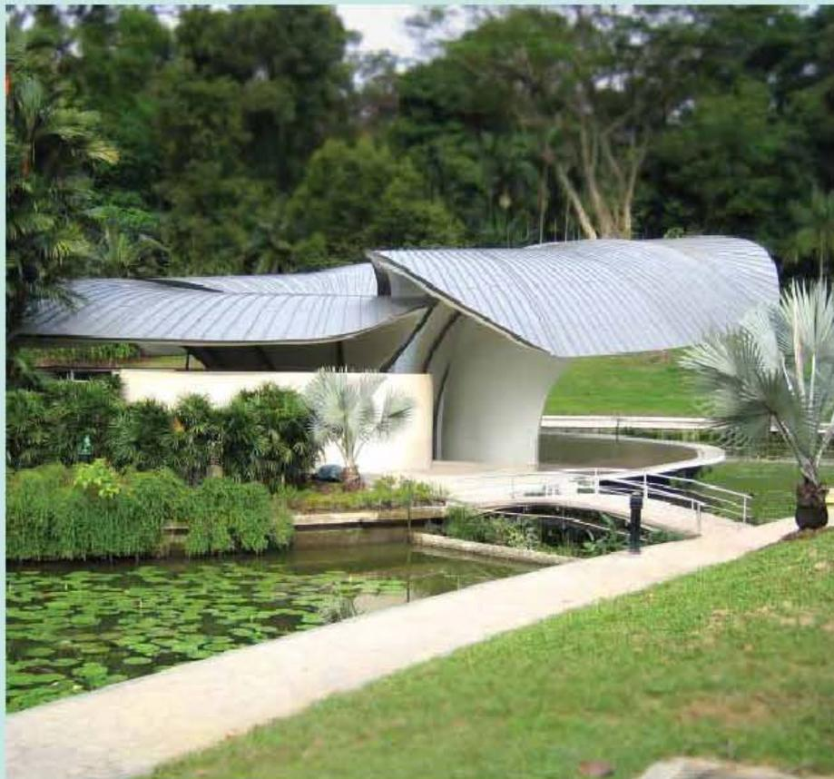
▲ The petal like form of the roof is constructed from free standing steel ribs that are expressed on the underside of the petals, and together with the ribbed form of the titanium zinc roof of above, evoke the complex venation of flowers and leaves. ▼
